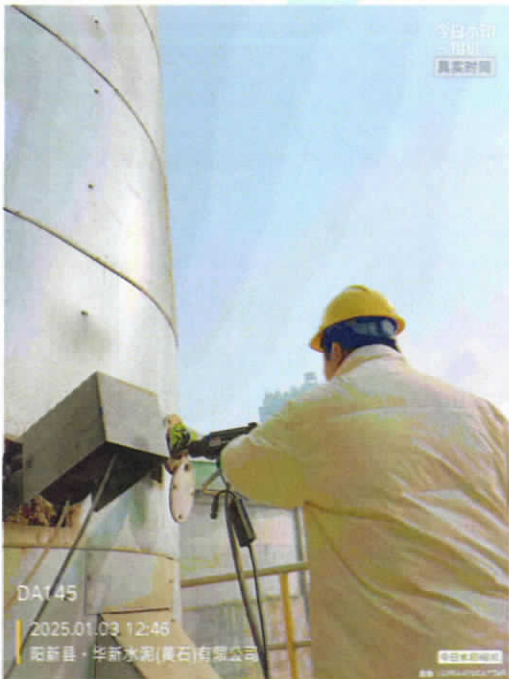
DA145 1#水泥磨辊压机废气排气筒采样口◎7
